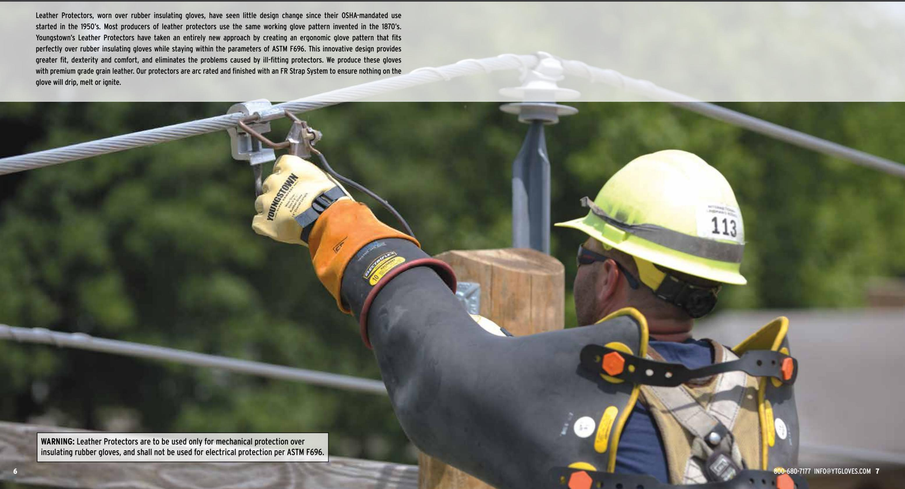
**WARNING:** Leather Protectors are to be used only for mechanical protection over insulating rubber gloves, and shall not be used for electrical protection per ASTM F696.
